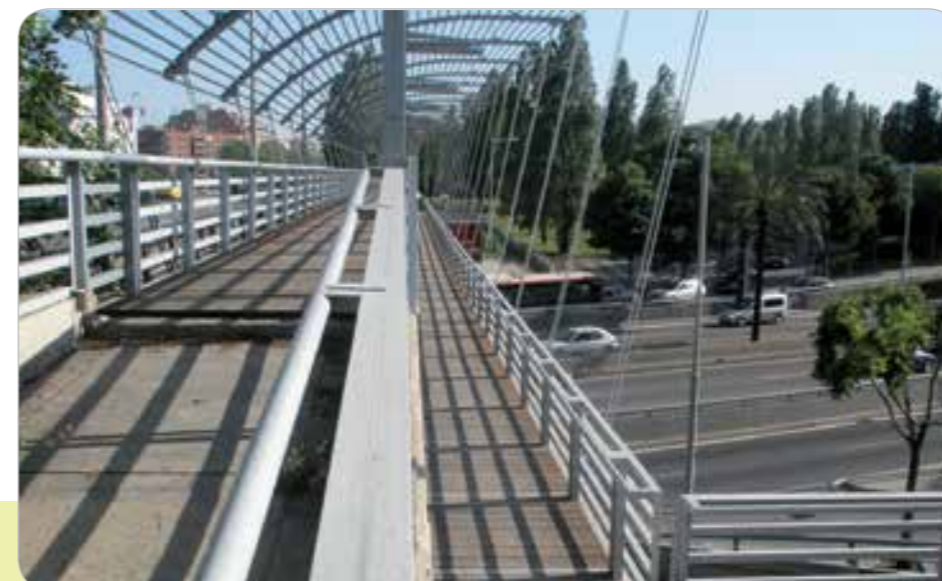
Pedestrian bridge over the highway leading to the southern districts
