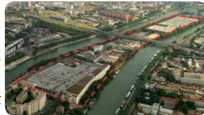
The industrial site along the river
